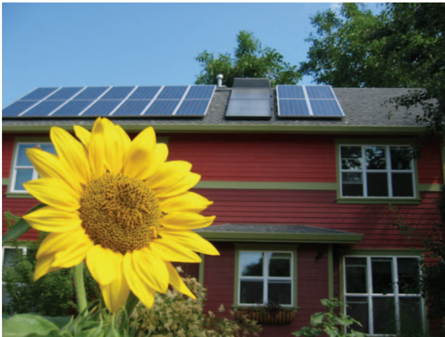
Source: Energy Trust of Oregon and Solar Oregon
